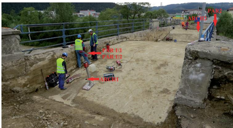
Fig. 3. The upper part of the bridge and notification of 4 sites for drilling bores
