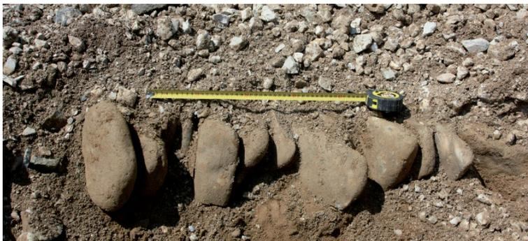
Fig. 2. Original bridge pavement found under the asphalt layer
