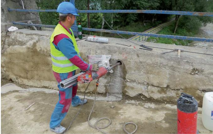
Fig. 7. Drilling the concrete core with diameter of 100 mm
